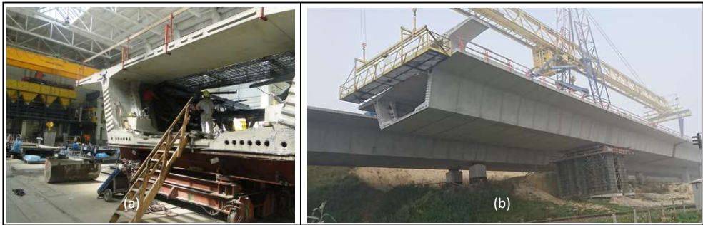
Fig. 7. Segments casting in in adjustable molds (a), self-launching truss gantry (b).
