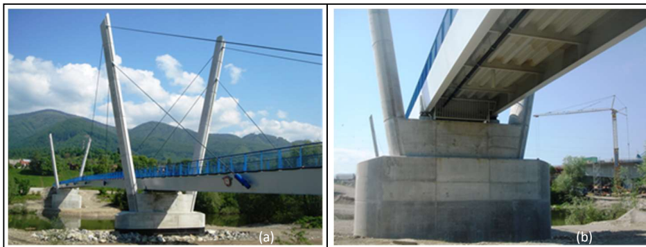
Fig. 4. Concept of tree spans cable-stayed footbridge (a) and components of orthotropic deck (b).
