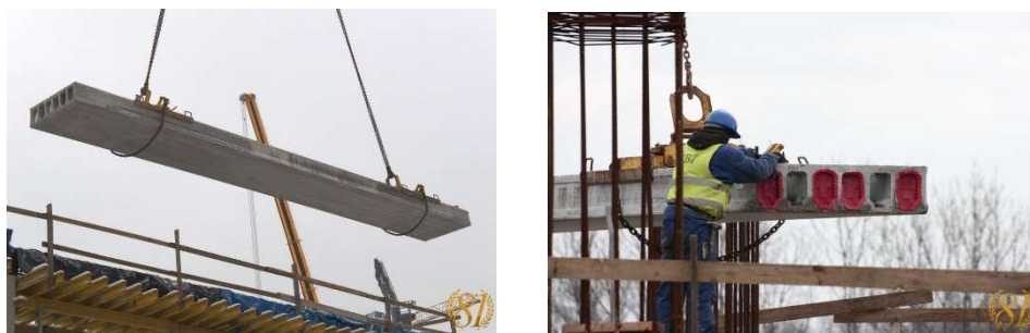
Fig. 1. Mounting the hollow core slabs [11].
