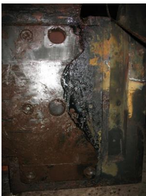
Fig. 1. Damages of lining strap of bottom WR chock from drive side (delivery side).
