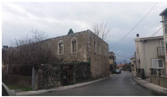
Fig. 23. Ruined facilities in Old Town today.
