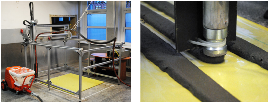
Fig. 1. Cartesian robot with pumping module during concrete printing.
