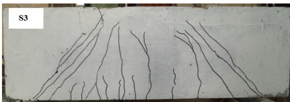
FIG. 6. CRACK PATTERNS COMPRESSION
