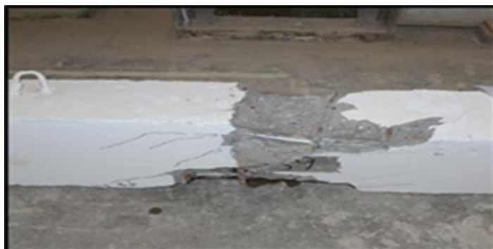
Fig. 14. Failure Mechanism of Tested Beam
