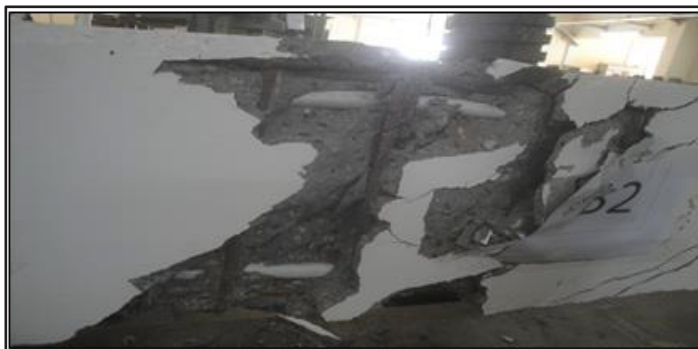
Fig. 13. Close-up Mode of Failure of Tested Beam
