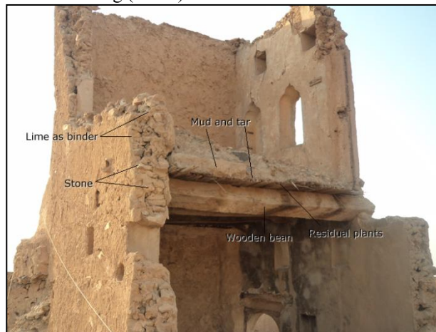
Fig.4. Walls and Roofing system in Hit Castle's houses
