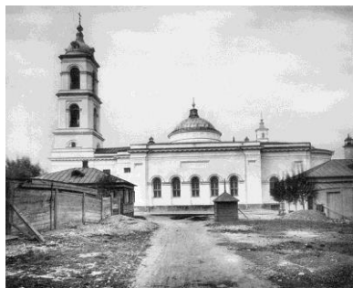
Fig. 2. The Church of Savior in Nalivki was demolished in 1929.
