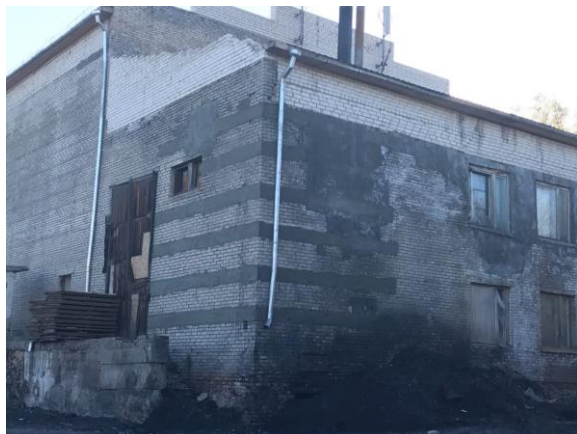
Fig. 7. The general view of the building after 4 years of operation
