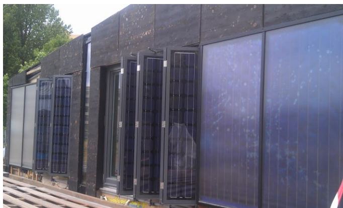
Fig. 3. An example of combining the functions of the protective screen and the photovoltaic element (PV) of the power supply system, implemented at the experimental facility of the energy-efficient building by staff and students of the University of Applied Sciences (HTW, Berlin, Germany. Photography from the personal archive of the authors).
