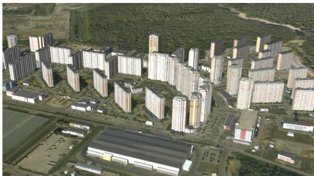
Fig. 1. 3D modeling of a typical residential area development, taking into account the transportation infrastructure and surrounding areas
