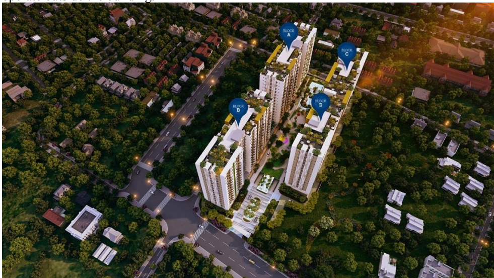
Fig. 1. Overall layout cannot be approached by fire trucks.
