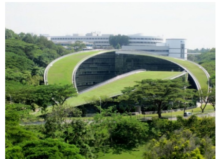
Fig. 2. Extensive green roof. [7]
