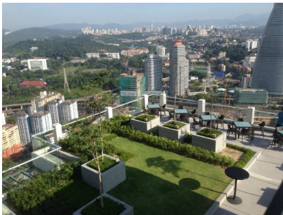
Fig. 1. Intensive green roof. [7]
