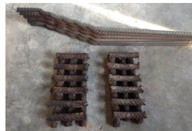
Fig. 4. Anchor bolt Pigtail and rig
