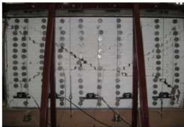
Fig. 3. Cracking pattern in the first specimen after 1.0 % in-plane drift cycles and arching phenomenon before failure under out-of-plane shake table motion
