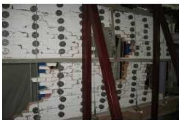
Fig. 4. Cracking pattern in the second specimen after 1.0 % in-plane drift cycles and partial collapse of masonry due to out-of-plane motion after 2.2 % in-plane drift cycles
