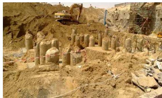
Fig. 1. Piles underneath the future Etisalat centre in Abu Dhabi
