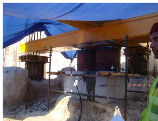
Fig. 4 Static Load test in the future Etisalat centre
