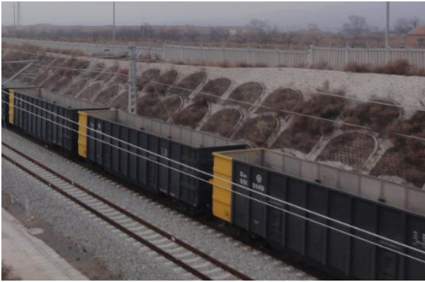
Fig. 1 Freight vehicle passing on ballasted track
