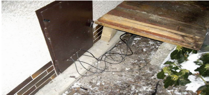
Fig. 1. View of probes placed in soil at family house structure.
