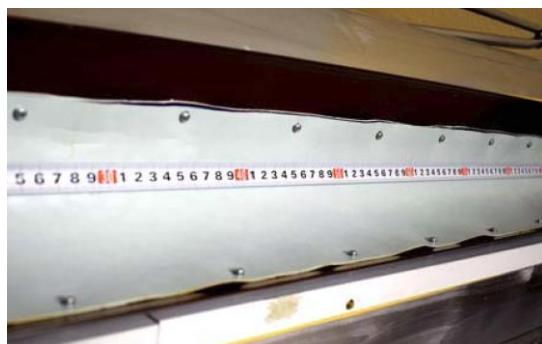
Fig. 5. Fragment of the experimental equipment with an open chute, and the applied coating Subcote FLP
