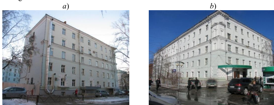
Fig. 1. General view of the building: northern (a), central and southern blocks (b).
