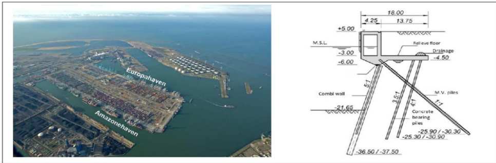
Fig. 1 Overview of the ‘Europees Massagoed Overslagbedrijf’ (E.M.O.) at the Amazonehaven (Left); Cross section of the quay wall at the Amazonehaven [10] (Right)
