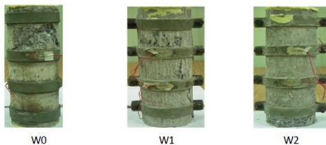
Fig. 12. Crack pattern of concrete cylinder S-10/30.
