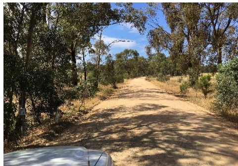
(a) S4 trial road section before stabilization
