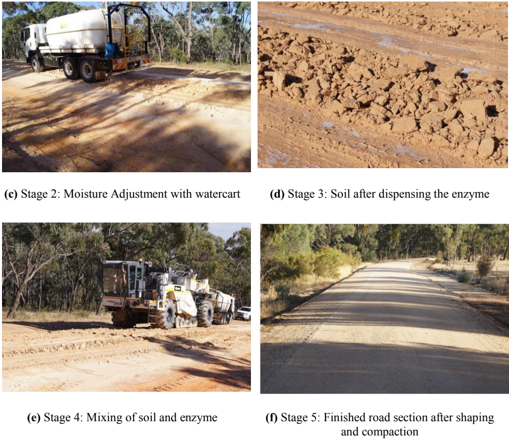
Fig. 3. Construction stages of trial road construction
