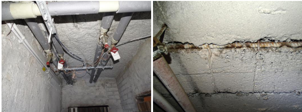
Fig. 5. Insulation of ceiling and ceiling with exposed reinforcement painted with the addition of gypsum (photos by Piotr Knyziak, 2016)
