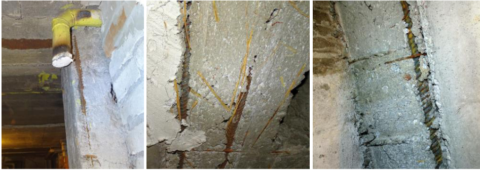
Fig. 6. No corrosion on reinforcement surface (photos by Piotr Knyziak, 2016)
