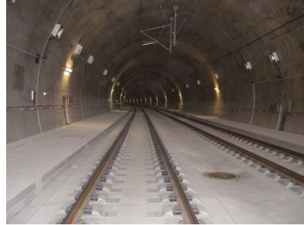
Fig. 3. Tunnel part of ballast-less track construction
