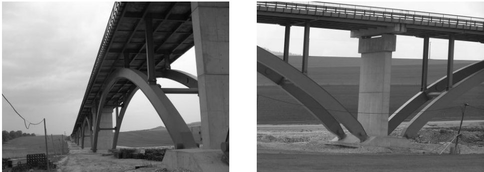
Fig. 3. Detail view of steel bridge arch and bridge support.
