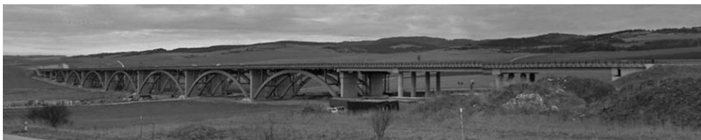
Fig. 1. General view of the bridge structure.
