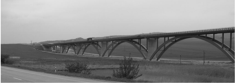
Fig. 2. View of steel bridge arch.
