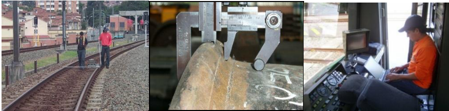
Fig. 12. The modernization work of maintenance services [4].
