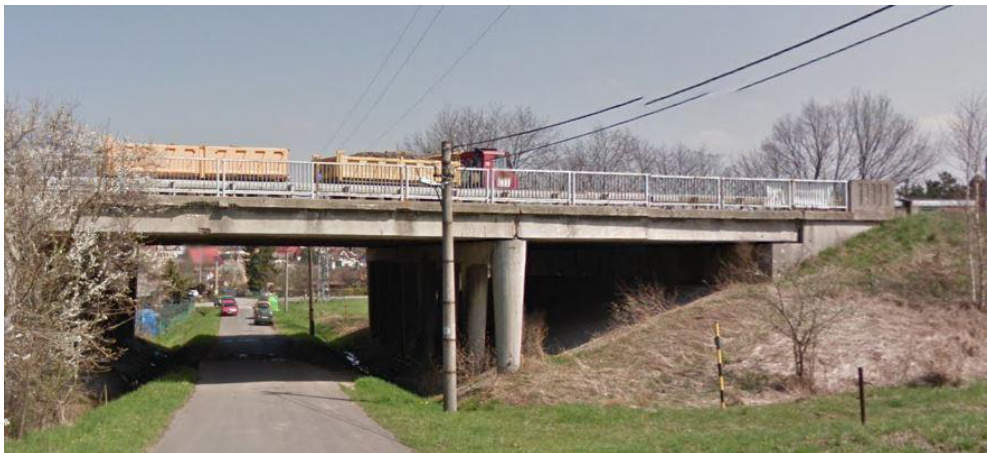
Fig. 1. View of the bridge structure.
