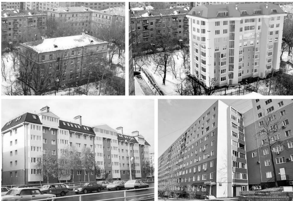
Fig. 2. Example of Reconstruction of Uniform Premises in Moscow (Before and After), Surgut and Vladivostok.
