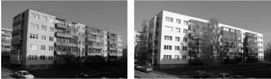
Fig. 1. Example of Modernization of the Soviet Period Building in Vilnius (Before and After).
