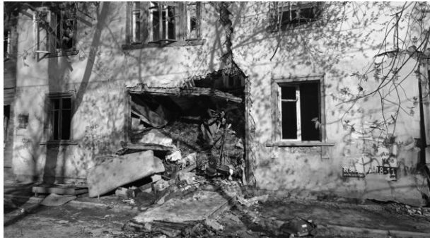
Fig.1. General view of a dismantled building and generated construction wastes
