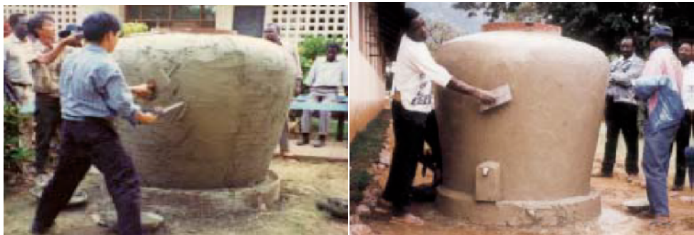
Fig. 2. Construction of 2,000-litre cement rainwater jar
