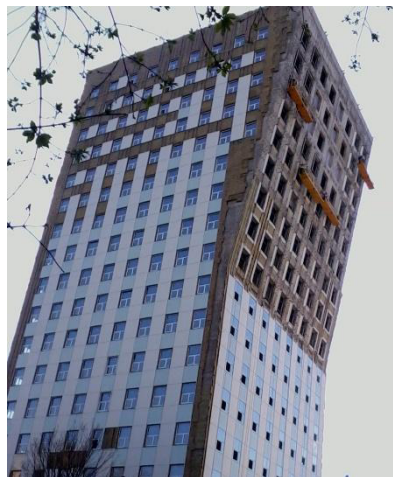
Fig. 3. Sloping with negative angle in the top part of building
