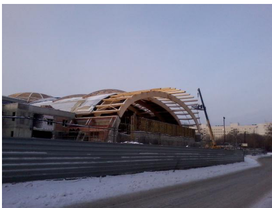
Fig. 4. Transfer workers on sport complex
