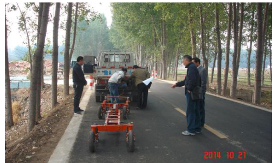
Figure 1. Pavement roughness testing in field
