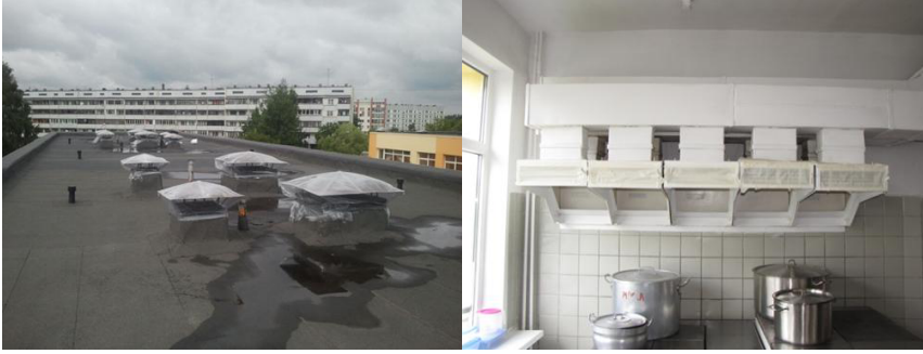
Figure 1. Preparation work for Blower Door test.
