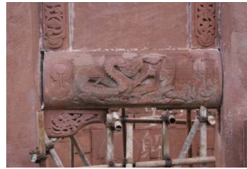
Fig. 4 The current situation of stone frames and QT construction
