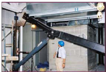
Damper installation in K-bracing
