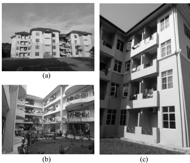
(a). Built-form configuration, enclosure and facade design - Large horizontal overhangs along the wall with windows, (b). Internal courtyard in the middle of residential building, (c). Casement and turn window design with tinted glass and large balcony in each residential unit faces to outside areas.
