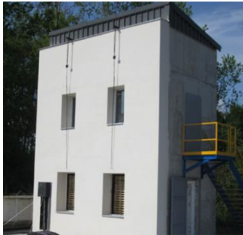
Figure 1. View of the Efectis LEPIR 2 facility.
