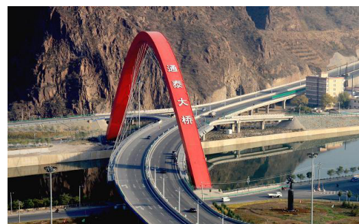
(a) Bridges photo
