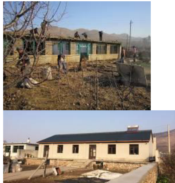
Figure 2. Exterior before and after Retrofit
