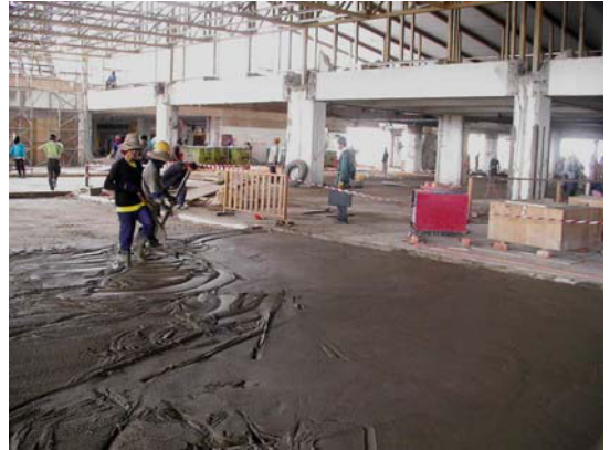
Figure 2. Slab thickening for airport project in Malaysia
