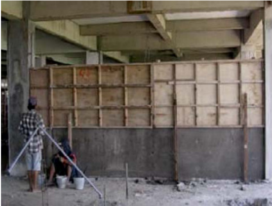
Figure 1. Cast in-situ wall in Surabaya, Indonesia
