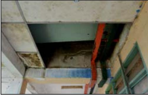
**Fig. 9:** Broken suspended ceiling
