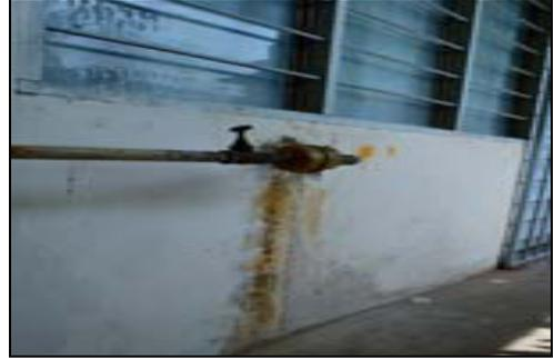
**Fig. 10:** Pipe leakage
