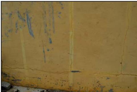
**Fig. 1:** Vertical and horizontal cracks on outer wall
