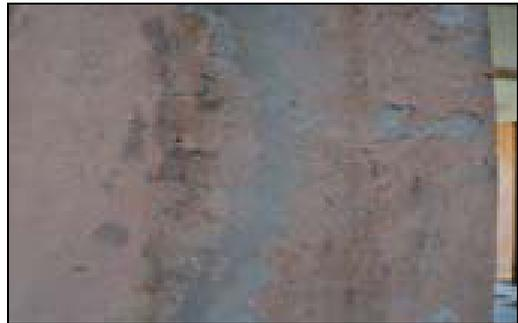
**Fig. 6:** Severely peeling paint on external wall
