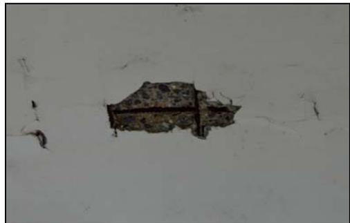
**Fig. 8:** Concrete spalling underneath the floor slab
