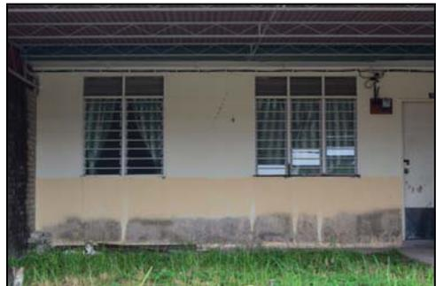
**Fig. 2:** Peeling paint on external wall
