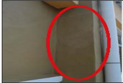
**Fig. 4:** Diagonal cracks on column area
