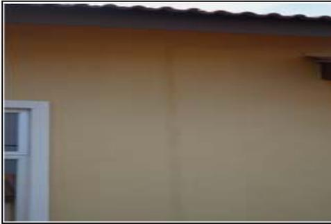
**Fig. 3:** Vertical cracks on external wall
