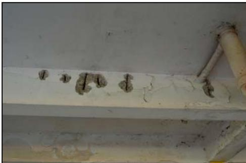
**Fig. 7:** Concrete spalling on beam area
