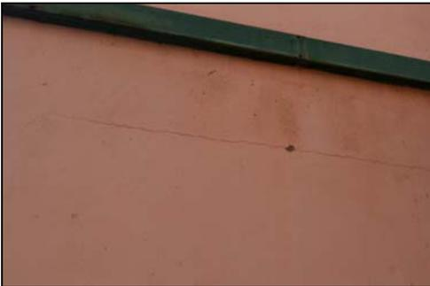
**Fig. 5:** Plaster cracks on external wall
