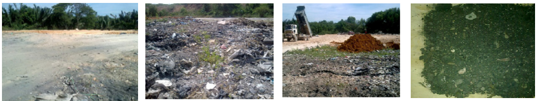
Figure 1: Teluk Kapas Landfill site
