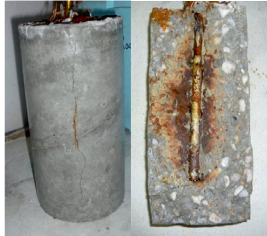
Fig. 4. Cracks on the material and corrosion of the stainless steel bar (28 day-treatment at 5 A/m 2 ).
