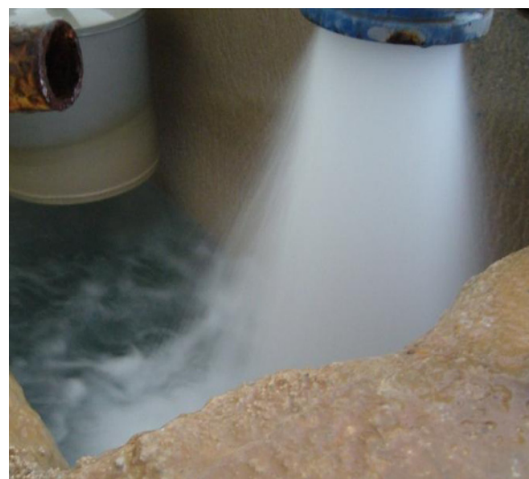
Photo 1. Photo of circuit breeze load of drinking water.
