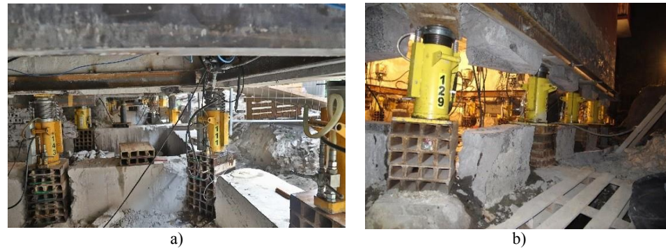
Fig. 11. Hydraulic jacks with piston fed from the central oil pump: a) jacks built into internal walls, b) jacks in the external wall.
