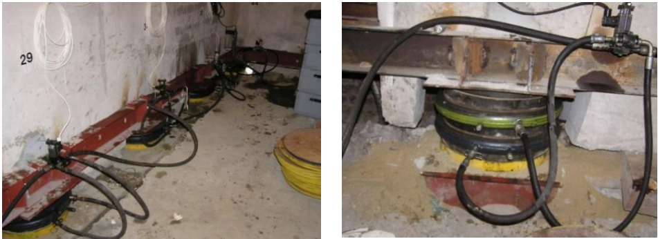
Fig. 7. Membrane jacks.
