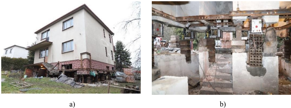
Fig. 9. A building during rectification: a) a photo, b) jacks in internal walls.
