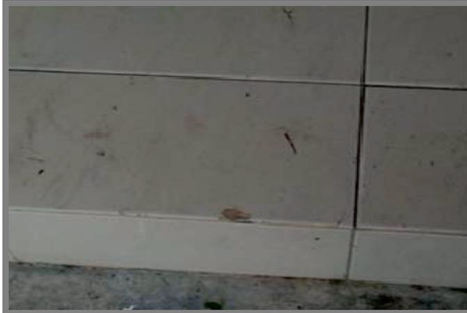
**Figure 8.** Broken tiles
