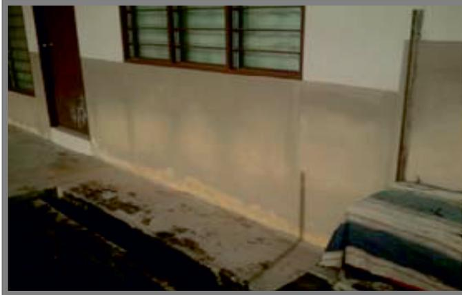
**Figure 5.** Discoloration on wall area
