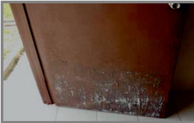
**Figure 6.** Peeling paint on door
